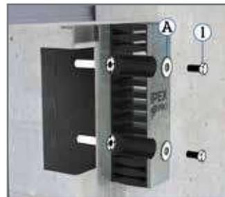
If there are no screw sleeves in the wall, the installation kit (bolt anchor) Order No.: BI-10038 can be used. The installation kit is available separately, see point 3.1 Additional mounting material.
